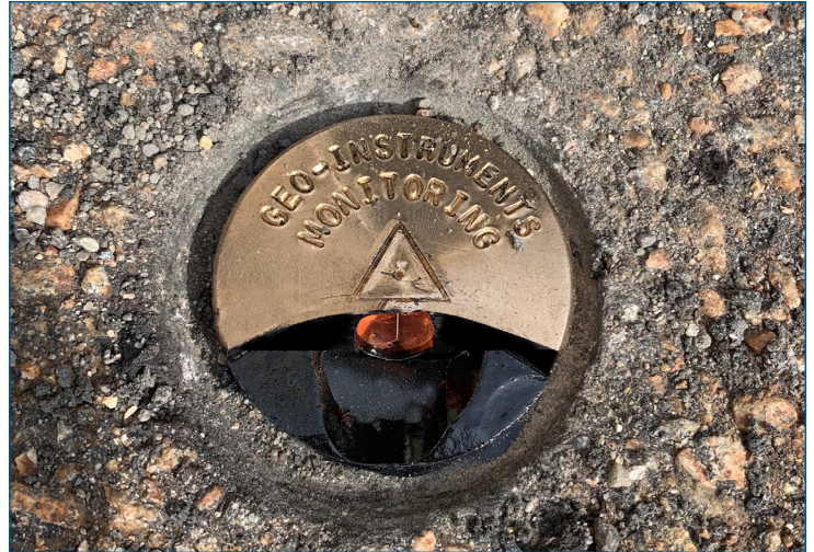
When fully grouted, the monument prism sits flush with the surface.
