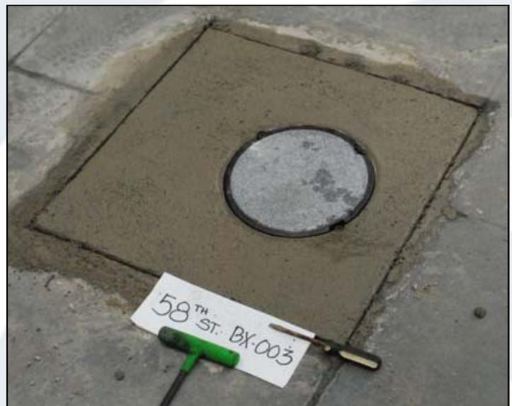
Inspection frame installed flush with grade.
