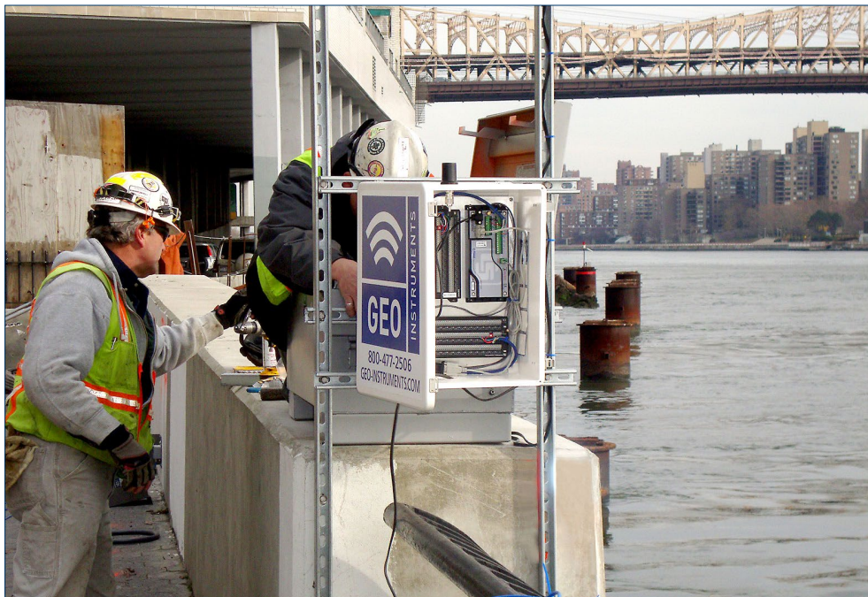
Installing a wireless datalogging system
