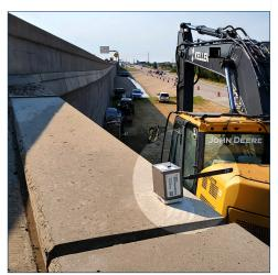
Wireless Tiltmeters monitor stability of MSE wall during major repair work.
