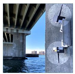
Wireless Laser-Tiltmeters monitor stability of bridge piers as bumper system is replaced.
