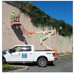
Wireless tiltmeters monitor stability of 40-foot retaining wall above public parking lot.
