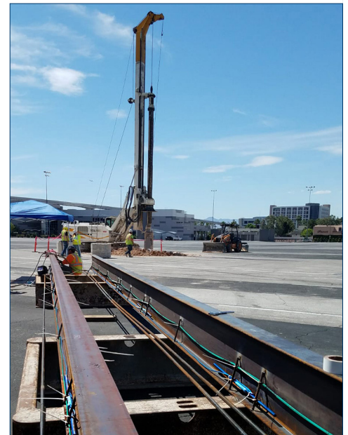
Sister bar strain gauges can be installed on H-beams using welded-on tie-points.
