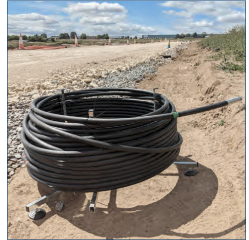
The profiler is pre-filled, sealed, and ready for installation. This eliminates deairing and flushing issues and the need for a reservoir.
