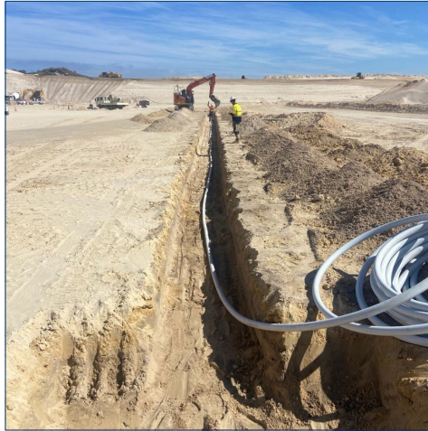
The automated settlement profiler has a range of 14 m and is available in lengths up to 125m. Sensors are spaced 1 to 5 meters apart.
