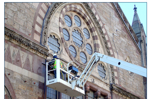
Old South Church Repair, Boston
