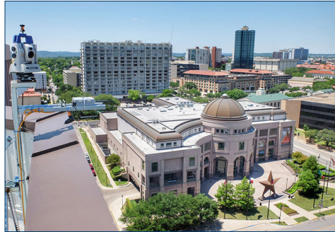
Capitol Complex Expansion, Austin
