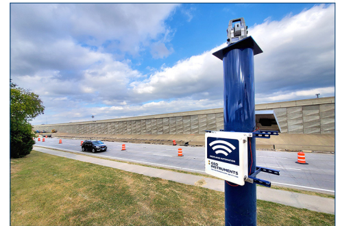
MSE Wall Repair, Texas
