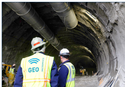
Bellevue Tunnel Construction, WA
