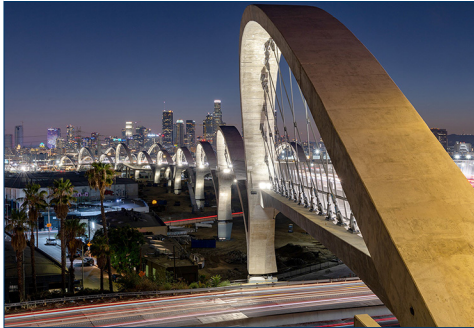
6th Street Bridge Construction, Los Angeles
