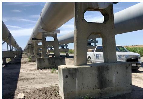
Mokulumne Aqueduct Retrofit, California
