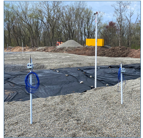
Settlement Plates and Piezometers
