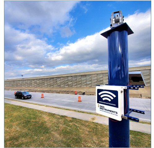
Monitoring was required during repairs to this MSE highway embankment.
