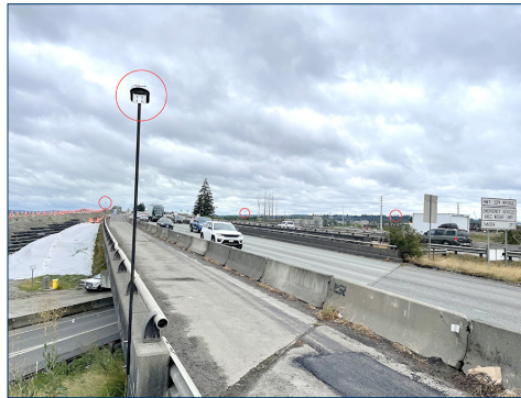
Highway bridge monitored for displacements during construction of new ramps.
