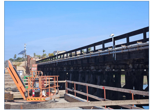
Rail bridge monitored for displacements during construction of replacement
