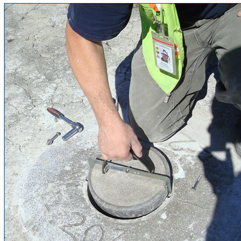
Placing the antenna in the finished installation.
