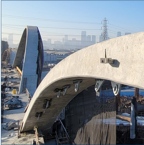
Laser-Tilt sensors monitored deflection of arches as they took on the load of the bridge deck.
