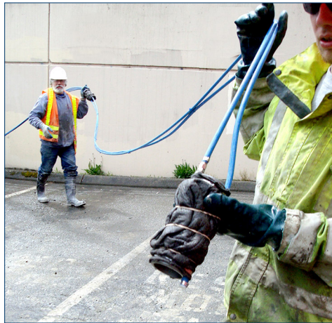
Installation of pre-assembled anchors and rods
