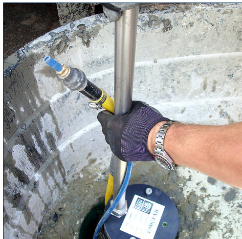
Installation of waterproof canister
