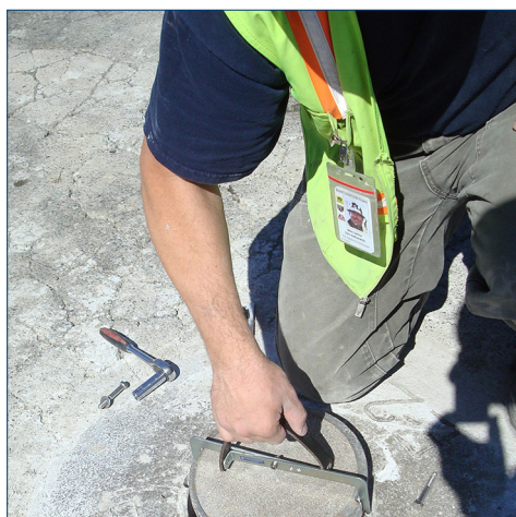
Installation of traffic rated Lid-Link® antenna
