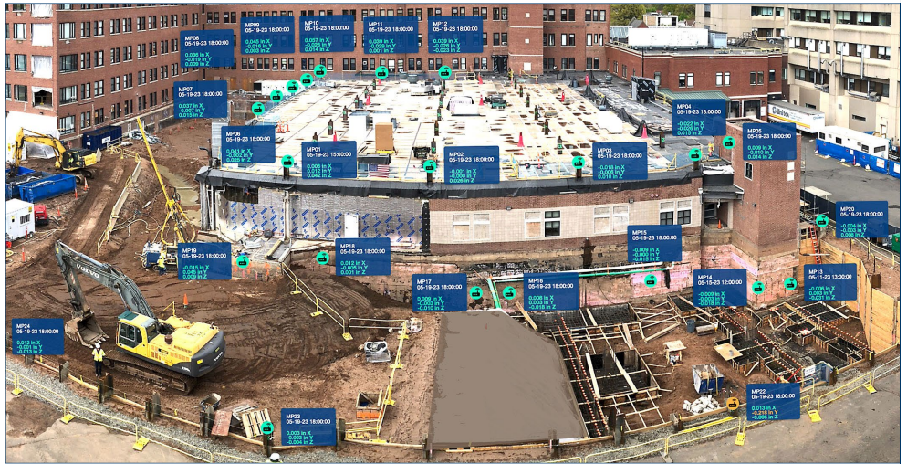
Planviews show sensors and readings superimposed on a base layer.
