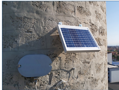
The AD-SIGNUM System provides automated asset monitoring for existing structures such as concrete bridges and dams. Sensors are compact, wireless, self-powered, and simple to install.
