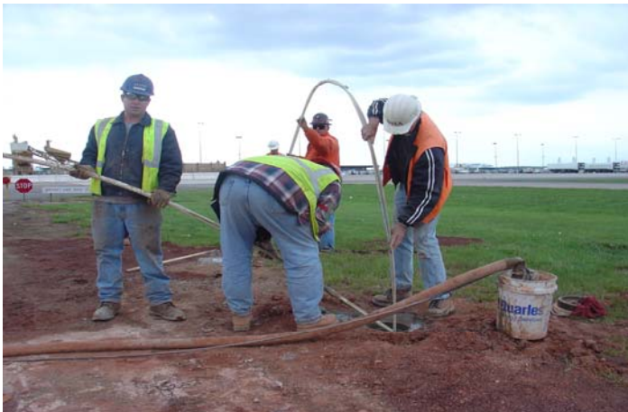
WMPBX installation insertion in borehole
