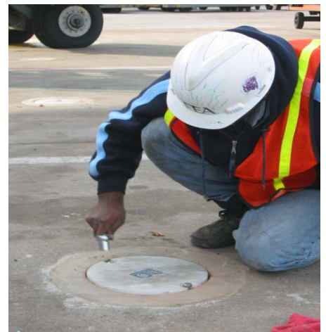
WMPBX head assembly installation at sur-
