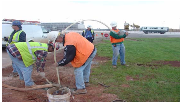
WMPBX installation insertion in borehole
