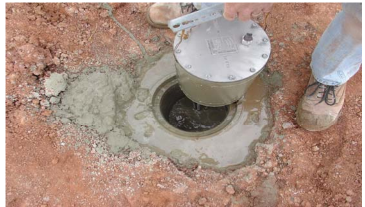
WMPBX head assembly installation at sur-
