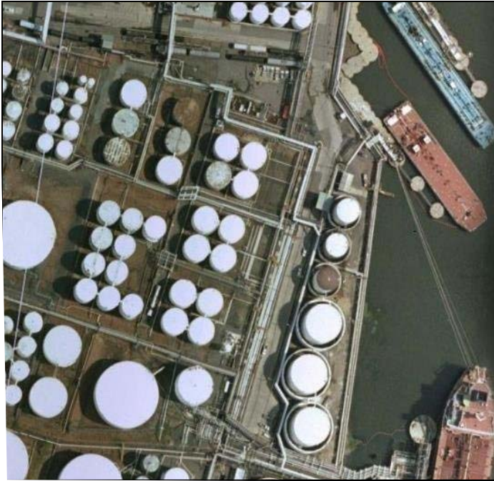
Above: Typical oil depot (tank farm) in use throughout the world.
