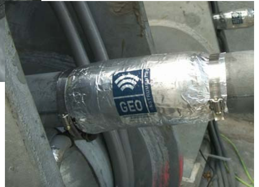
Above: Applying neoprene rubber protective layer. Right: Complete installation, with aluminum layer
