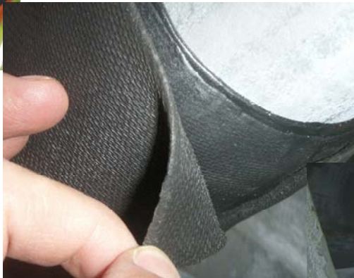
Above: Applying neoprene rubber protective layer. Right: Complete installation, with aluminum layer
