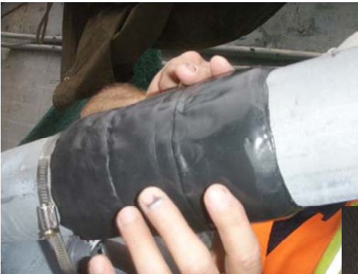
Above: Applying secondary gage waterproofing rubber.
