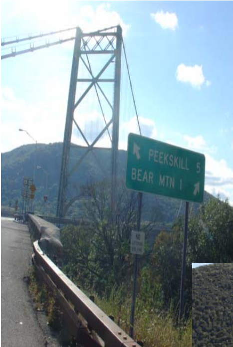
Above: View of the East tower on the bridge
