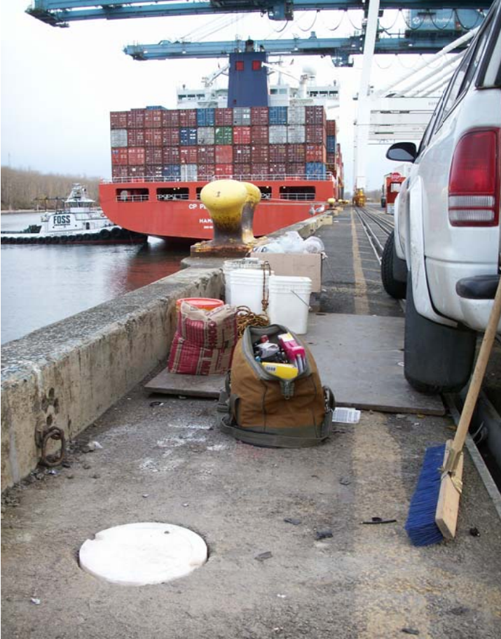
Right: Completed flush mount logger system, below: Flush mount SS lid, and flush antenna (upside down), below, foreground weldments for load cell bearing.
